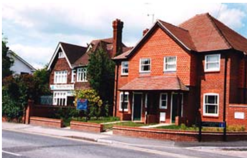
17. New development in the village, Pangbourne Place 18 houses and flats, 2/3 storeys, on site of former garage in village centre: hipped roof, gable, canopy, hanging tiles, bricks, in keeping with neighbours.
