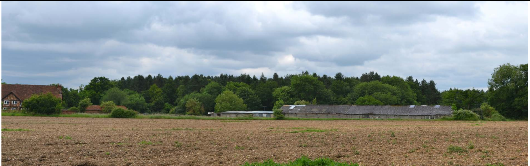
Viewpoint 1: View south to the site from the footpath to the north on the edge of housing south of Conifer Drive. Vicarage Wood behind the site.
