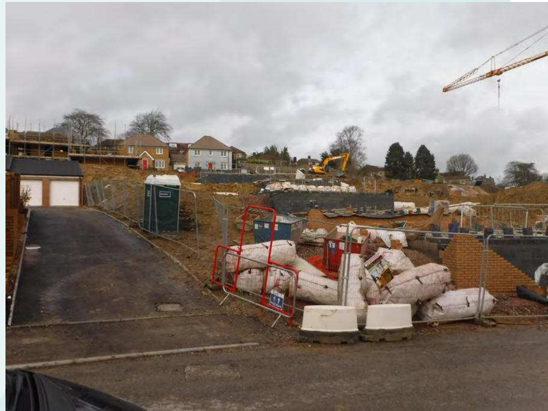
Construction site (© JBA Consulting)
