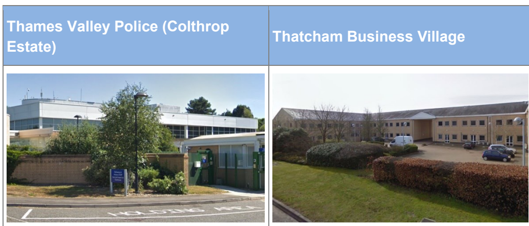
Figure 4.6 Office space in Thatcham
