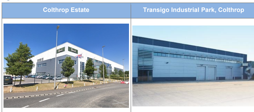
Figure 4.16 Industrial space in Thatcham
