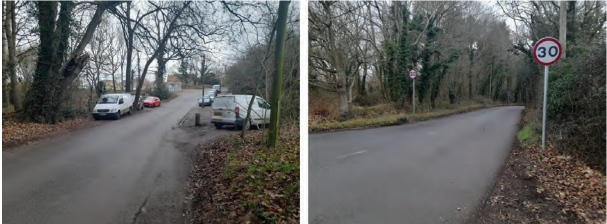
Figure 8 – Long Lane Site Frontage
