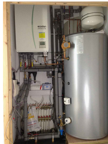
TYPICAL HEAT PUMP ARRANGEMENT (INTERNAL)
