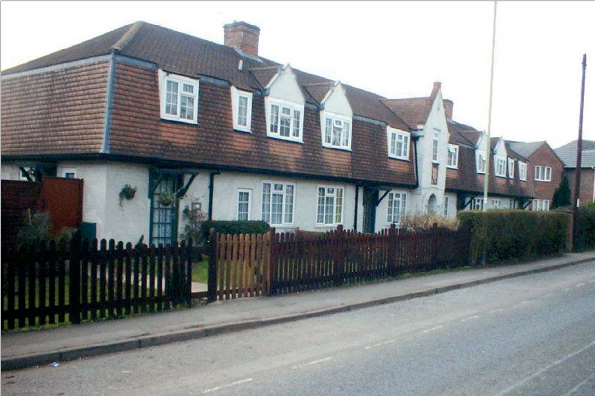
Plate 21: HUCA 41: Mill Lane - Terraced houses
