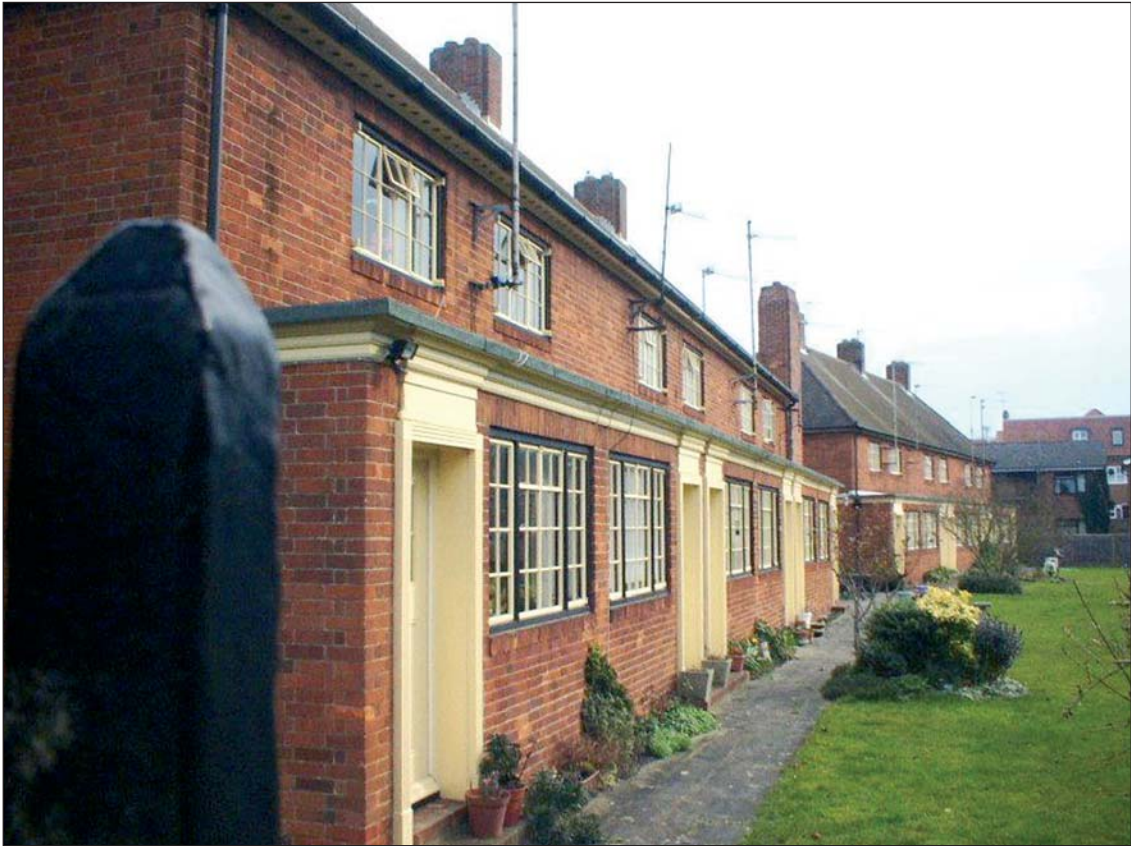
Plate 7: HUCA 10: Oddfellows Road - John Kimber almshouses
